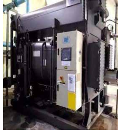
An absorption chiller and biomass boilers were installed to reduce the impact of climate change
