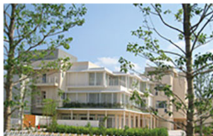
Domyoji-Takadonoen, a general-purpose welfare facility
